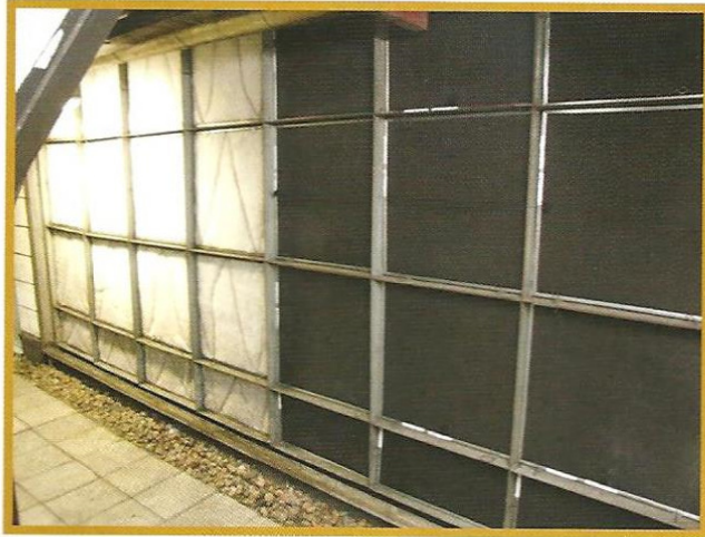
Disposable white polyester filter media tested on the left, PreVent® washable electrostatic Model R filters on the right.
