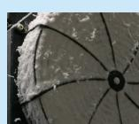
**PreVent filters** are a simple solution, affixed to the outside of an air intake, for easy access and fast maintenance.
