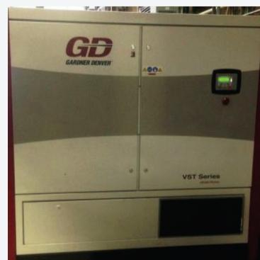
Equipment air intake openings located at foot traffic level are prone to pull in dust and debris along with necessary fresh air.
