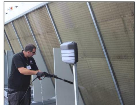
Installation began by cleaning the coil fins, 64 in total, with a pressure washer and water to remove grime and protect aluminum fins from chemical damage.
