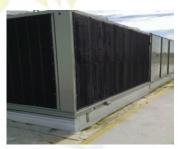
100 ton Trane Unit AFTER with durable, cleanable PreVent air filter screens
